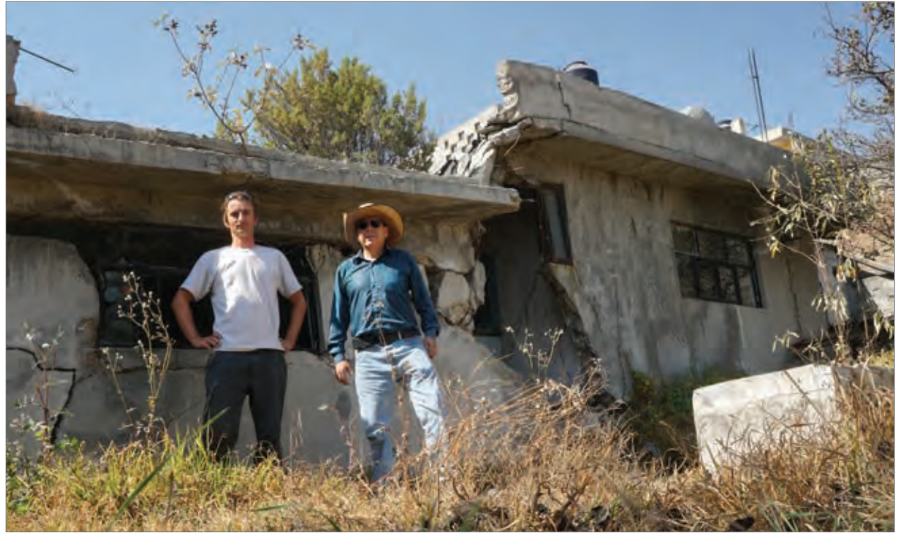
Pascal Castellazzi and colleague Jaime Garfias stand in front of an abandoned house in Toluca Valley, Mexico. The house is located along a fracture showing differential movement of up to 5 centimeters (2 inches) per year. (Courtesy P. Castellazzi)
