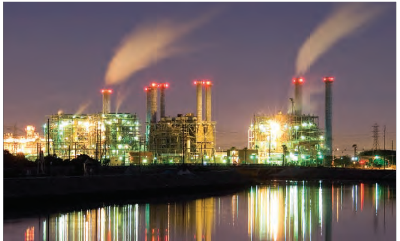
A full moon illuminates this power plant near Seal Beach in Rossmoor, California, not far from Los Angeles. (Courtesy alkhodarev/flickr)
