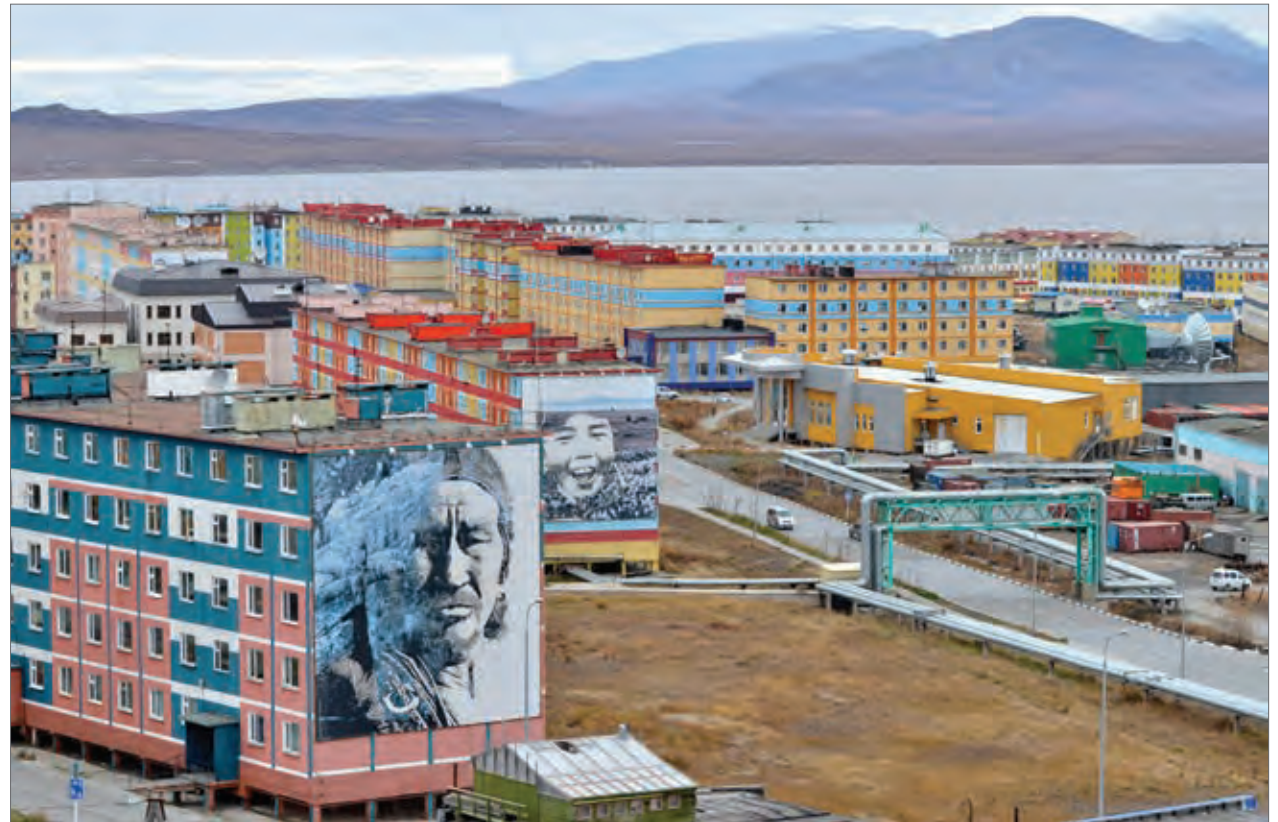
These buildings in Anadyr, Russia, are built on foundation piles to prevent heat from thawing the frozen ground below. (Courtesy US Consulate Vladivostok)
